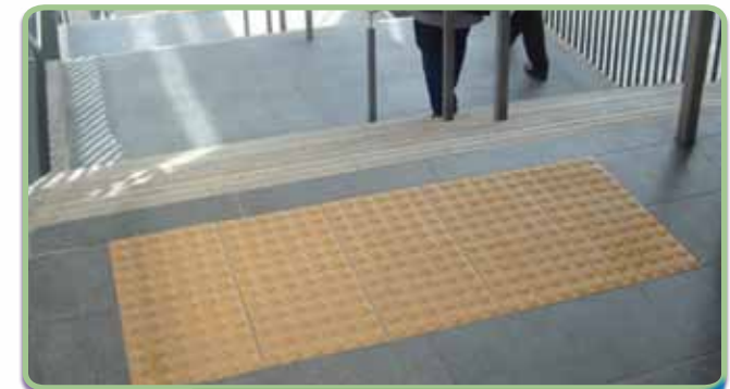
Figure 8 – A tactile wayfinding surface indicating a change in level
