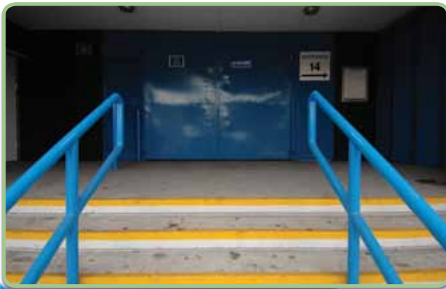
Figure 9 – Colour contrasting on steps
