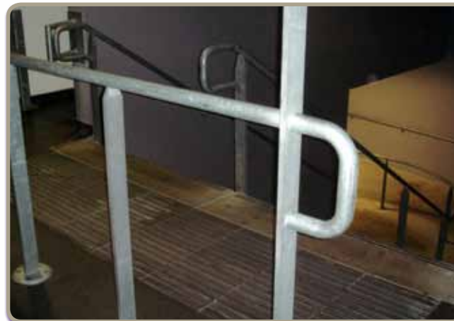
Figure 16 – Tactile paving (detectable warning) with a barrier at the top of the stairs
