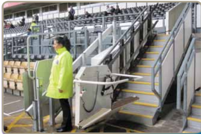
Figure 13 – An external, non-enclosed stairlift at Pride Park, Derby County FC, England
