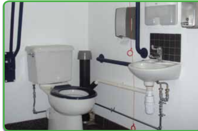
Figure 24 – An example of an accessible toilet
